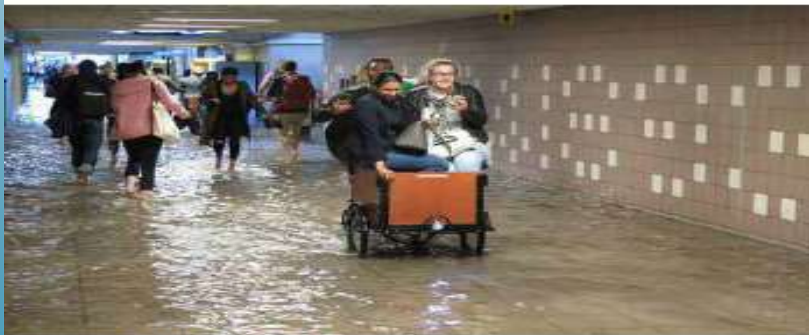
opmerking: overlast, tunnel Hollandspoor
